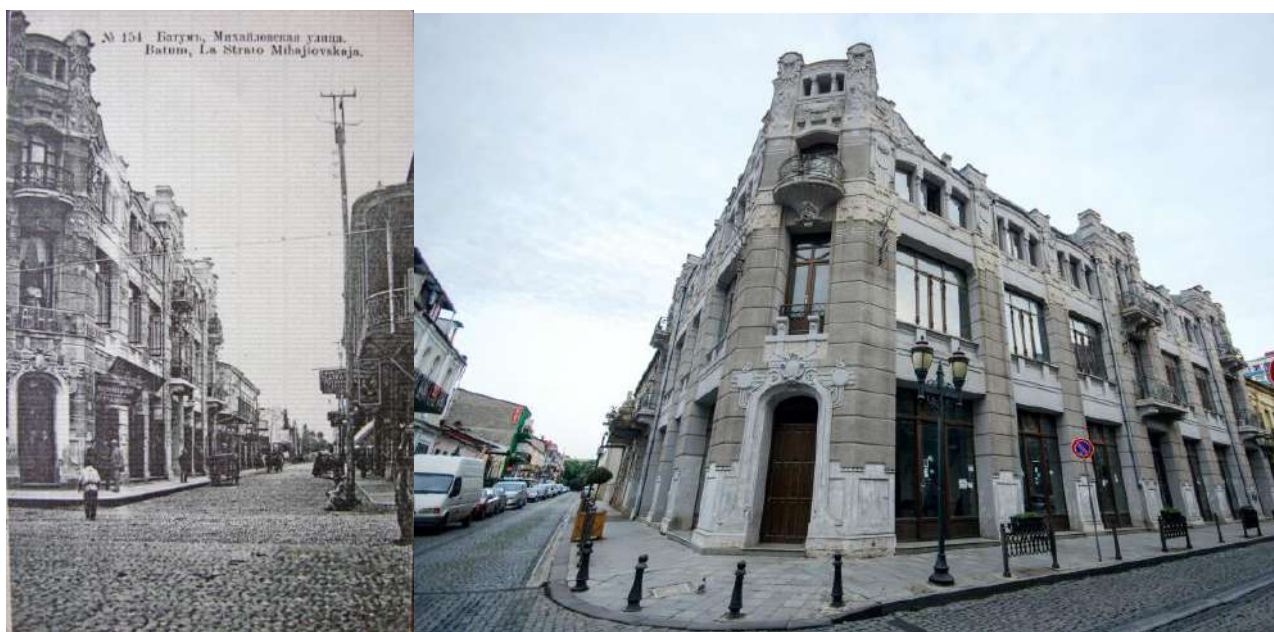
Building at 14 Zviad Gamsakhurdia Street, Batumi
