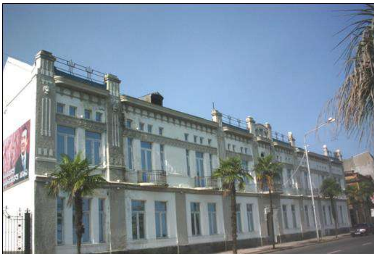
Building at 16 Iakob Gogebashvili Street
