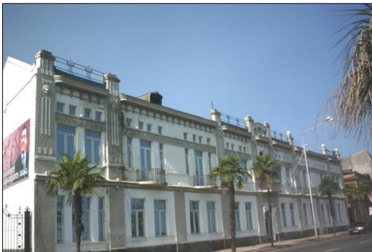
Building at 16 Iakob Gogebashvili Street
